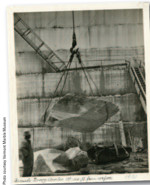
Historical Photo: Lifting a slab of marble 110 feet at the Vermont Marble Company
