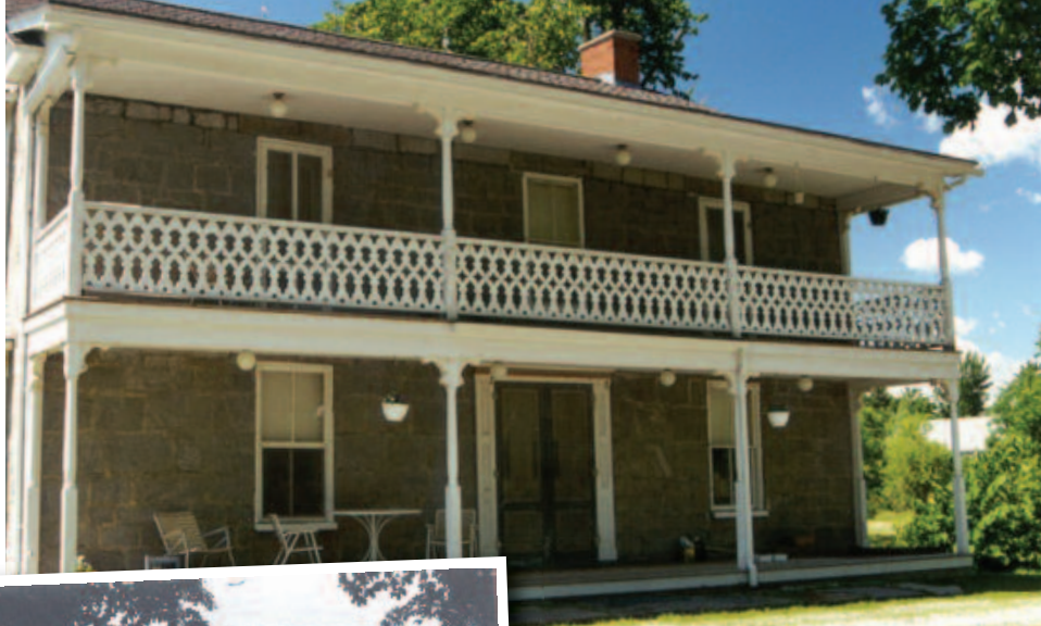
Ira Hill House, Isle La Motte
